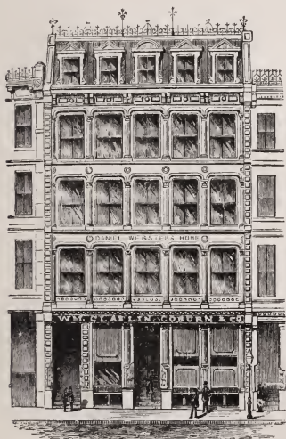
Site of Webster's Home, Summer Street.
